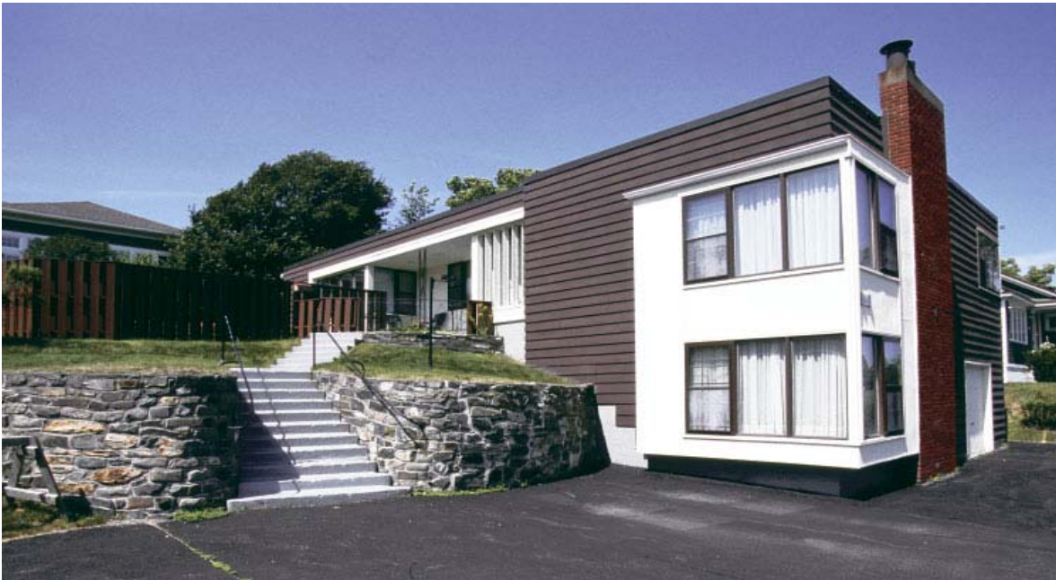
Figure 26: The Clouston Residence, designed by architect F. A. Colbourne in the early 1950's.
