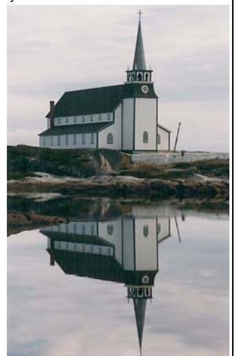
The restoration of St. Luke's Anglican Church, Newtown earned the Town of New-Wes-Valley a Southcott Award from the Newfoundland Historic Trust in 2006.
